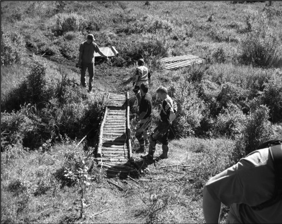
Rocky Mountain Dirt Riders Association Project - Single track upgrades in progress.
