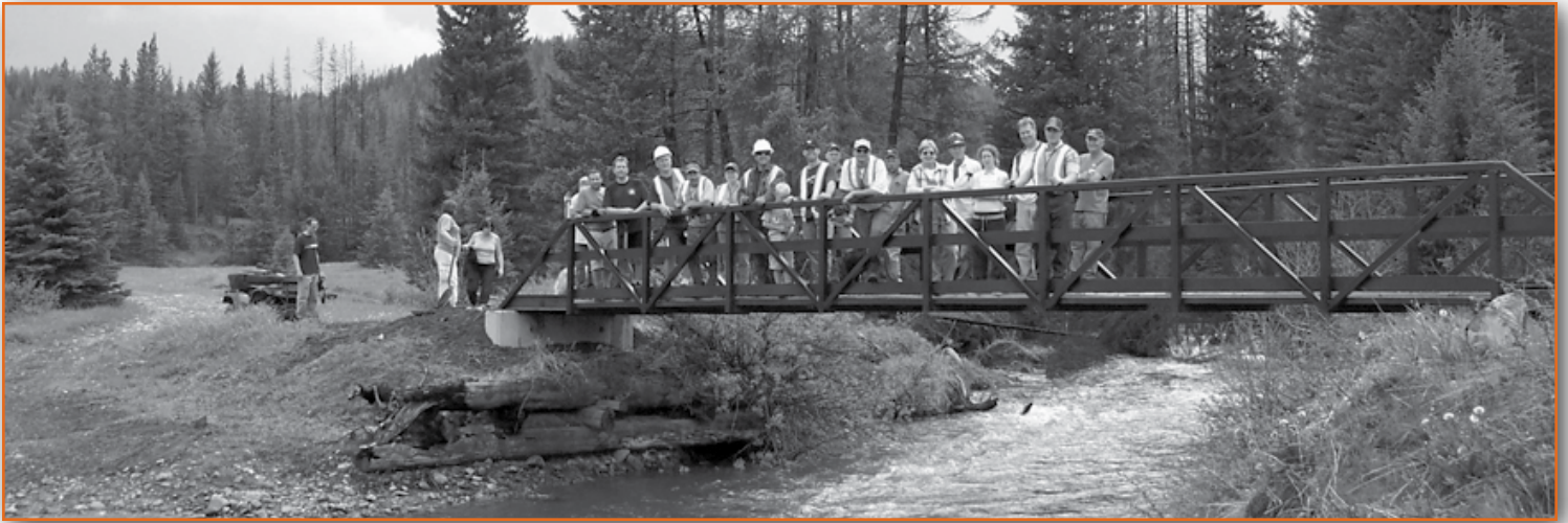
One of the many bridges being upgraded by Crowsnest Pass Quad Squad volunteers.
