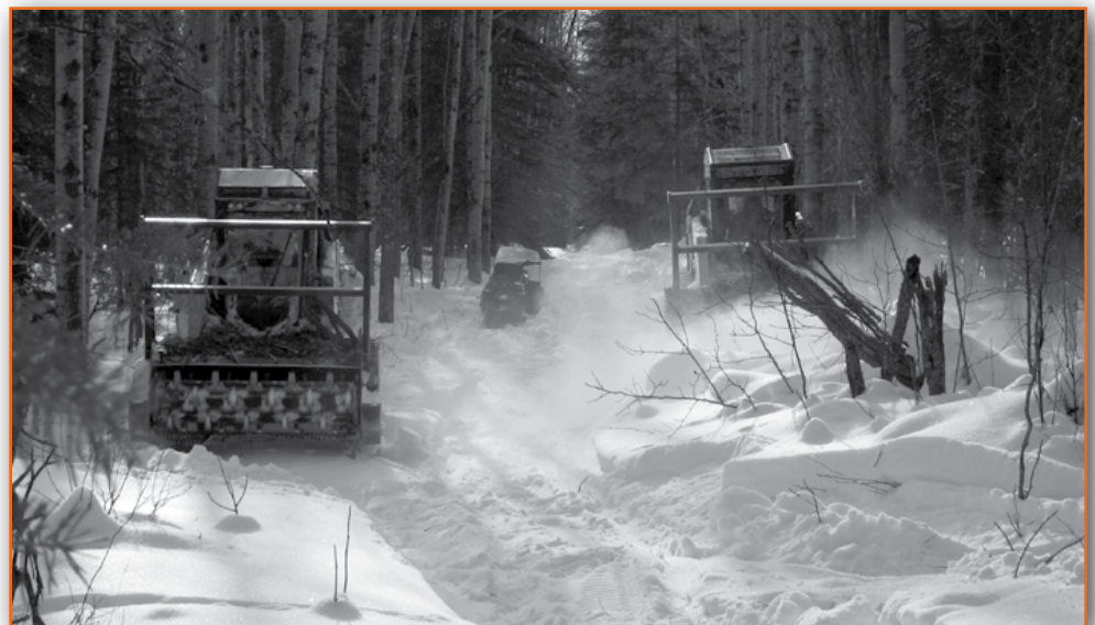
Construction underway on the Peace River Trail.
